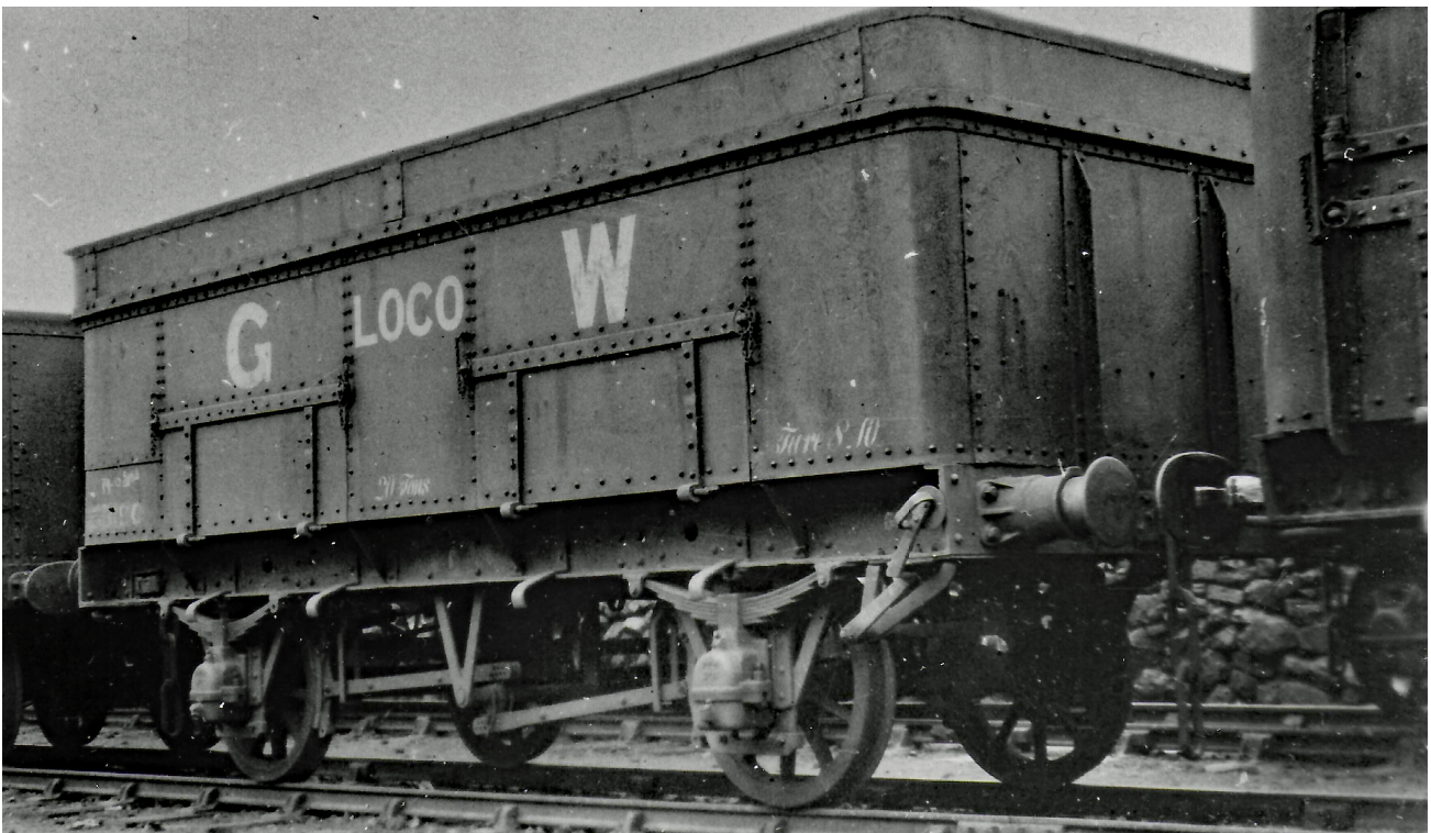
20 ton Loco Coal wagon with the number to the bottom left (unfortunately unreadable), "20 Tons" centrally and Tare 8-10 to the bottom left. HMRS M14732
